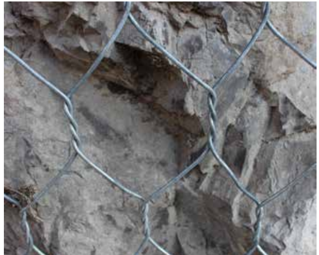
Rock fall net protection net laid in Sogno (BG)
