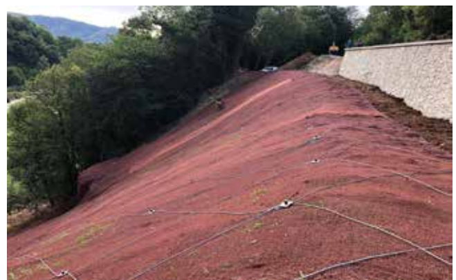
ArrMat brown cortical strengthening on mixed slope
