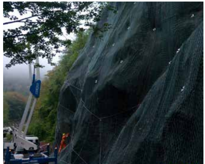
ArrFort Pet geocomposite laying phases
