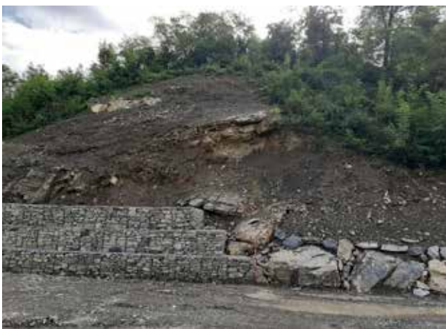
Pre-intervention underslope Ferriere situation
