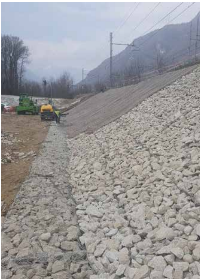
Railway under-slope coating - Domodossola (VB)
