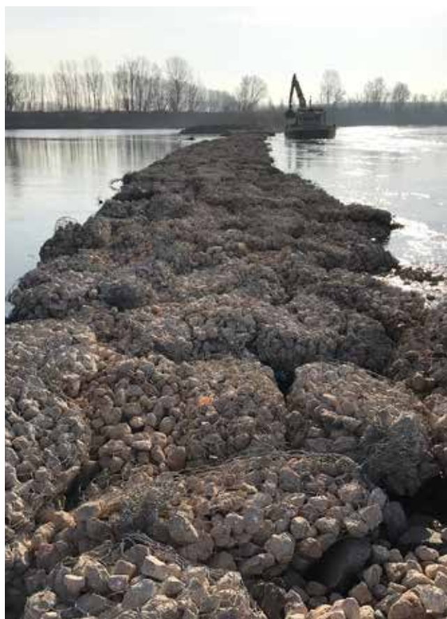
Paintbrush in sack gabions - River PO Torre d'Oglio
