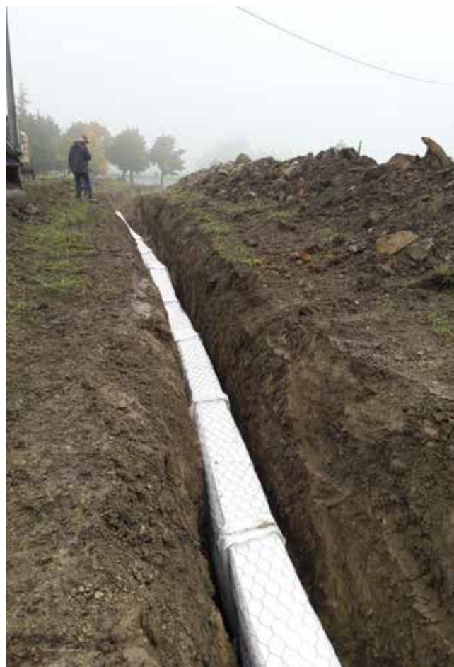
Drainage in agricultural ground - Loc. Costa Rustigazzo (PC)
