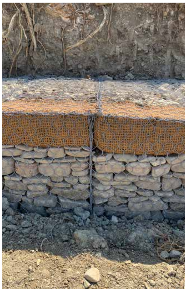
Greening gabions with vegetative pockets - Pavia
