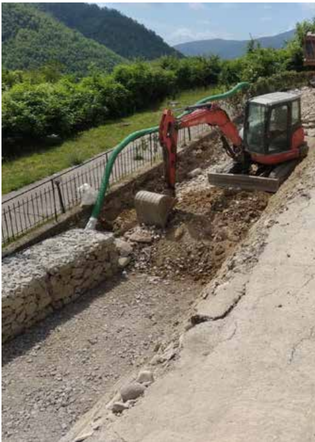
ArrSystem system, road under-slope consolidation -Podenzana (MS)
