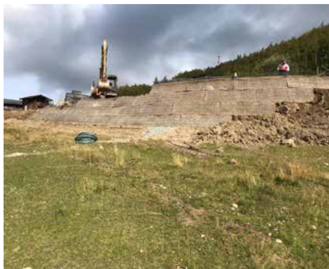
Embankment for new ski under slope - Sestola (MO)
