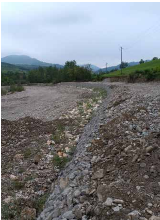
Bank defense in cylindrical gabions - Lugagnano (PC)
