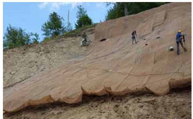
Arco installation phase - Valle Castellana (TE)
