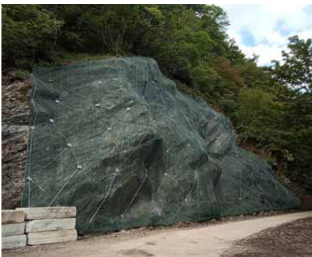
Reinforcement completed with ArrFort Pet - Fopla of Solignano (PR)
