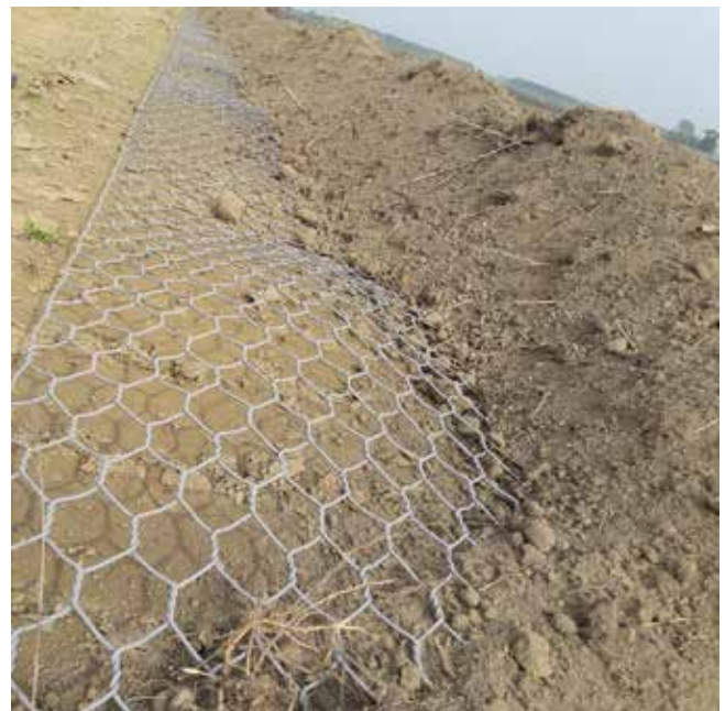
Anti-coypus net coating with scotic ground
