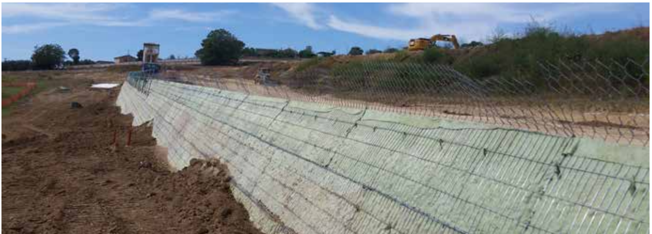
New road embankment for access to the Fermo hospital
