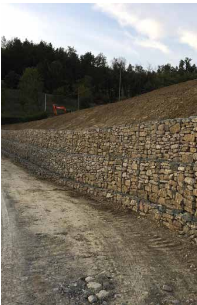
Road bank work-Travo (PC)
