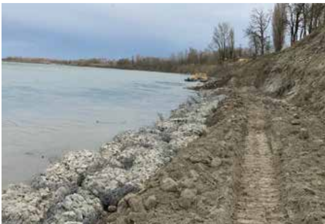
Bank defense in sack gabions - River PO Torre d'Oglio
