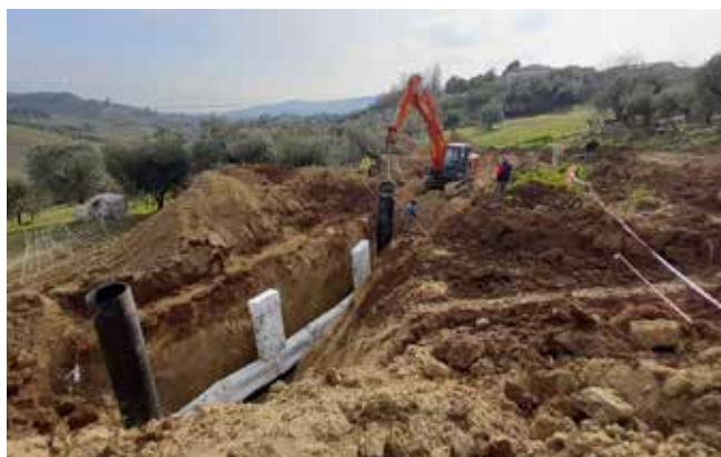
Laying of the drainage section - Tortoreto (TE)
