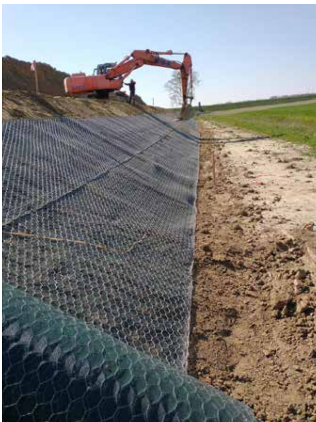
Embankment laying of the anti-shamber and anti-erosion net - Rottofreno (PC)
