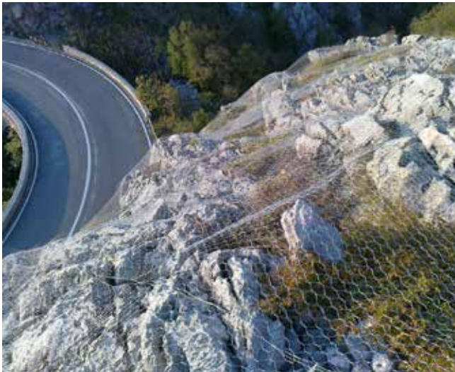
Rock fall net protection net laid in Croatia
