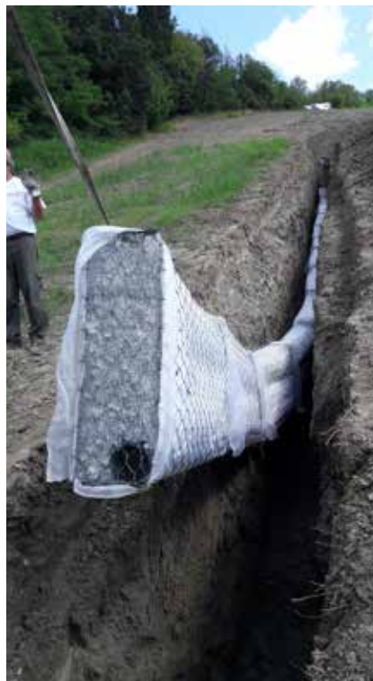
Draining trench with forced section on the ski slope - Veneto
