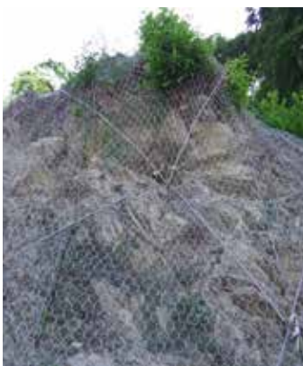
ArrMet for slope strengthening in fractured rock - Genoa
