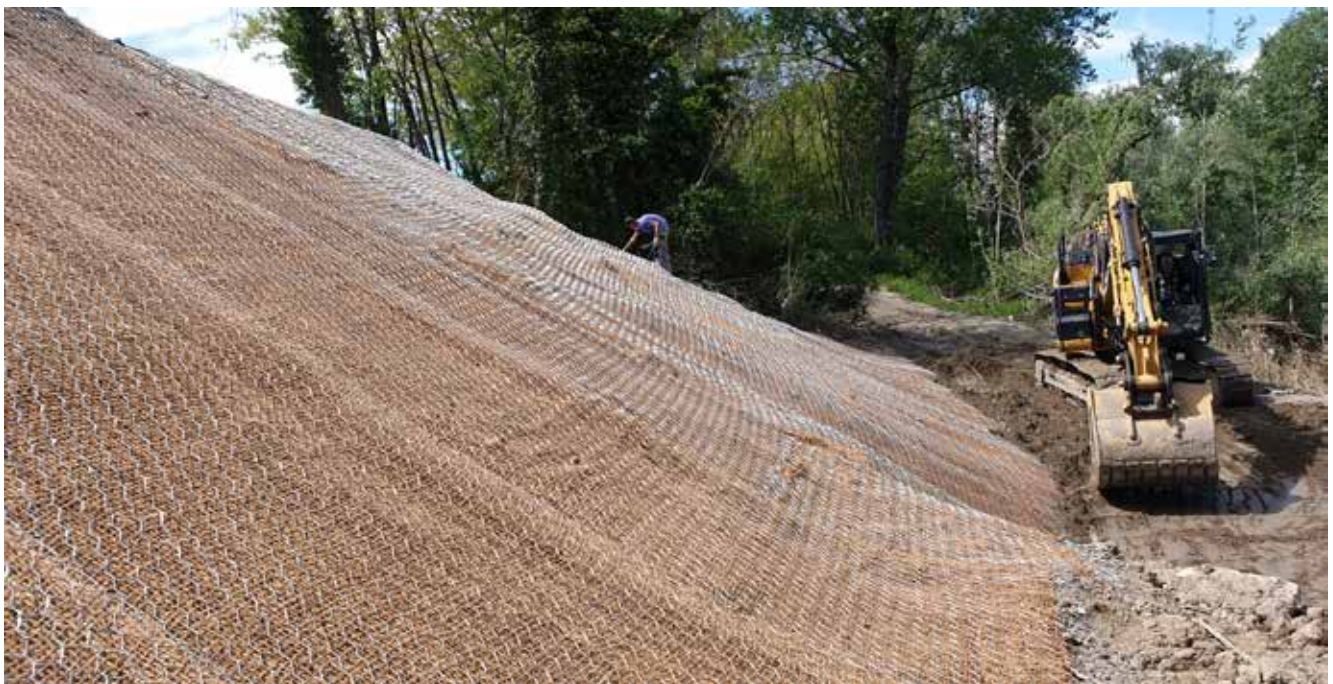
Low impact embankment and anti-coypus coating - Mantua
