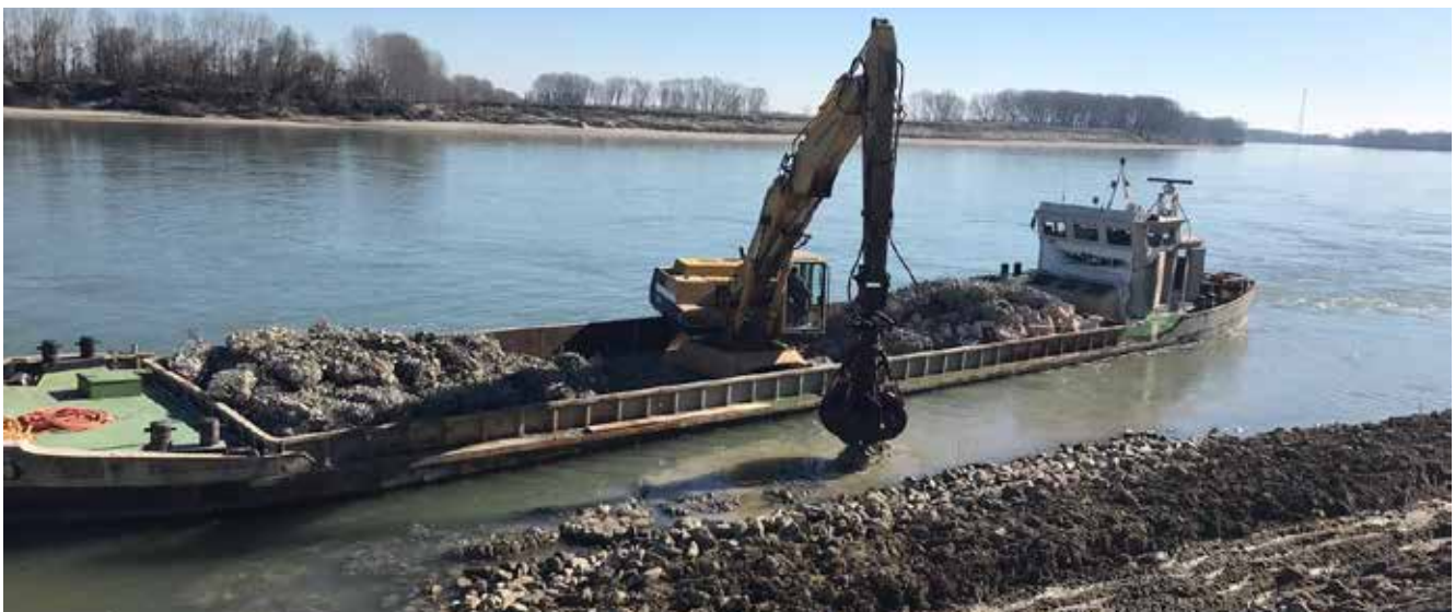
Laying of sack gabions from barge - River PO Torre d'Oglio
