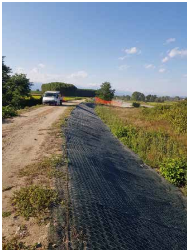
Anti-erosion and anti-shamber net to embankment protection
