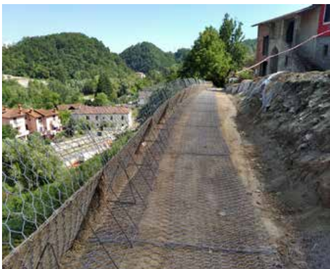
Road widening and slope consolidation - Pontremoli (MS)
